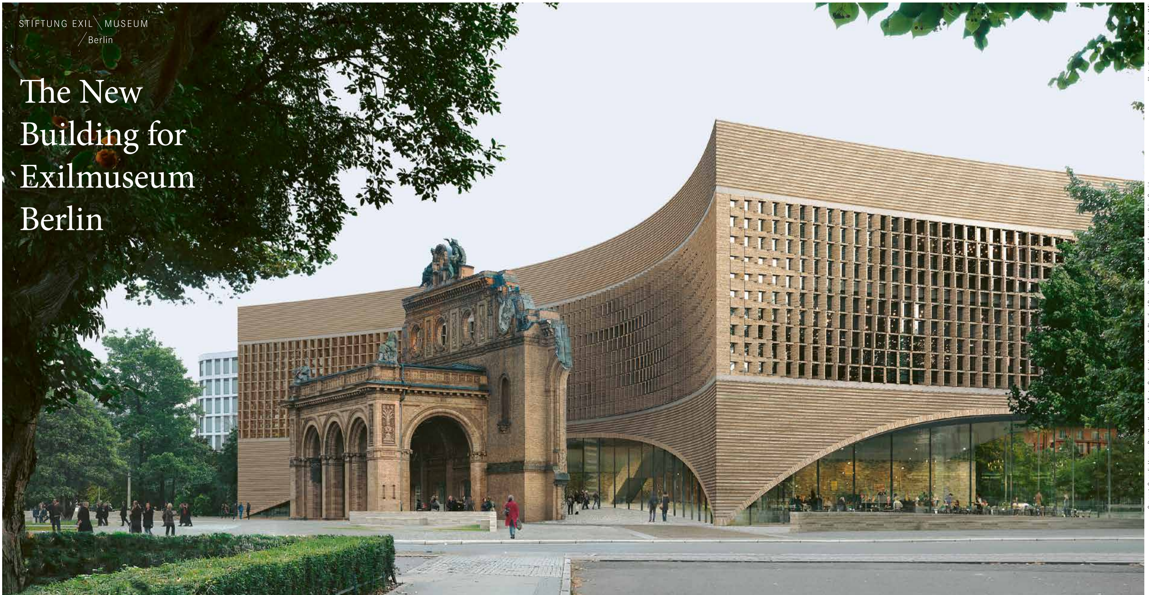
Illustrations: Dorte Mandrup/Mir Concept: Cornelia Vossen, Dorothee Käser / Texts: Cornelia Vossen, Sarah Blendin / Design: Dorothee Käser / Translation: Brian Currid
